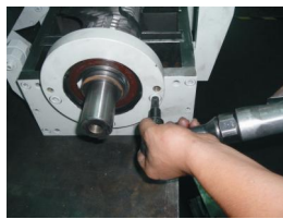
Picture 3-5: Installation of Bearing and Blade Rest 1 3
