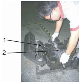
Picture 3-4: Installation of Bearing and Blade Rest 2
