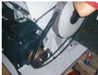
Picture 3-6: Installation of Belt and Belt Pulley 3
