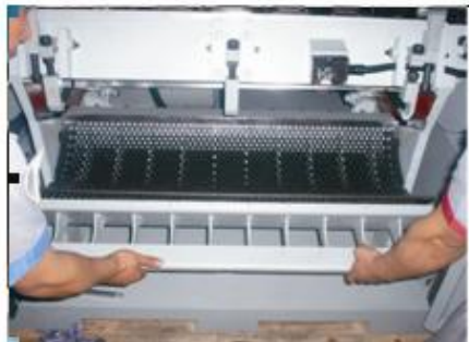
Picture 3-10: Installation of Screen Bracket and Screen
