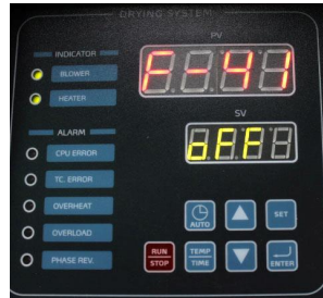
Picture 4-13: Reaction Time of Low-temp. Alarm
