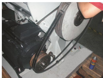
Picture 3-6: Installation of belt pulley and motor 3
