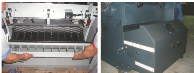
Picture 3-10: Installation of regrind storage bin, screen and screen bracket
