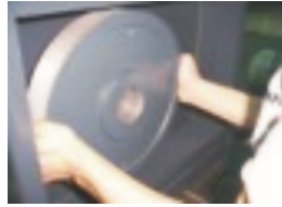
Picture 3-5: Installation of Belt and Belt Pulley 2
