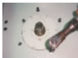
Picture 3-4: Installation of Belt and Belt Pulley 1
