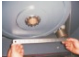
Picture 3-9: Installation of Belt and Belt Pulley 6
