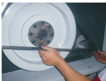
Picture 3-7: Installation of Belt and Belt Pulley 4
