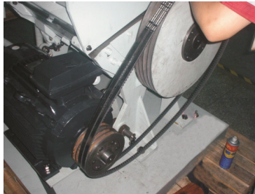
Picture 3-6: Installation of Belt and Belt Pulley 3
