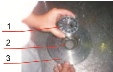
Picture 3-2: Installation of Bearing and Blade Rest
