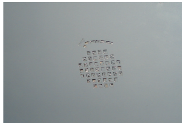
Picture 4-1: Check the Running Direction of the Blower
