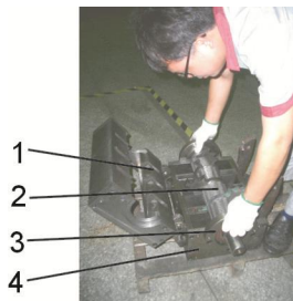
Picture 3-4: Installation of Bearing and Blade Rest 2
