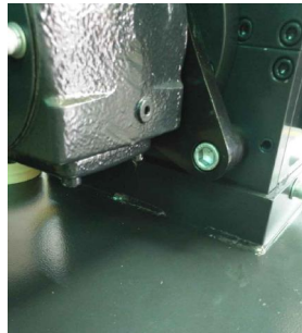
Picture 3-6: Installation of Motor 2
