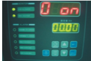
Picture 4-3: Intermittent Running Setup 3
