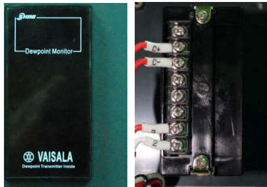
Picture 6-12: Connection of Signal Wire
