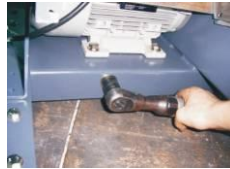
Picture 3-18: Installation of Belt and Belt Pulley 8
