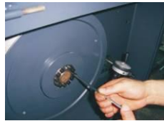
Picture 3-14: Installation of Belt and Belt Pulley 4
