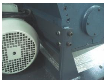
Picture 3-28: Installation of Material Collection Box 3
