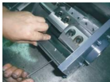
Picture 3-10: Installation of Rotating Blade and fixed Blade 4
