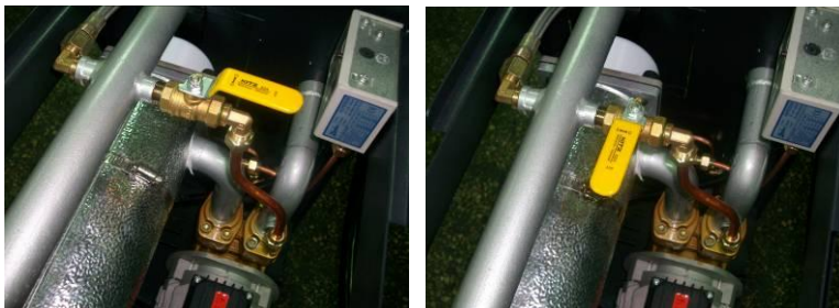
Picture 6-8: By-pass Globe Valve
