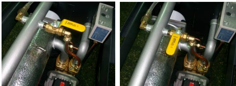
Picture 6-8: By-pass Globe Valve
