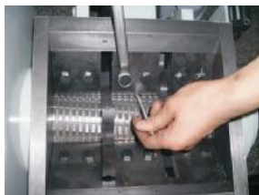
Picture 3-9: Installation of Rotating Blade and Fixed Blade 3
