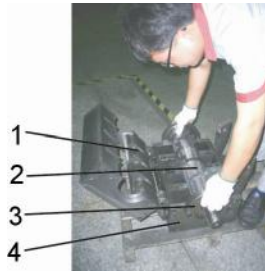
Picture 3-4: Installation of Bearing and Blade Rest 2
