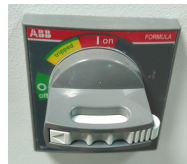
Picture 4-2: Main Power Switch
