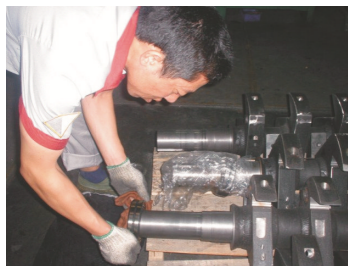
Picture 6-4: Installation of Bearing and Blade Rest
