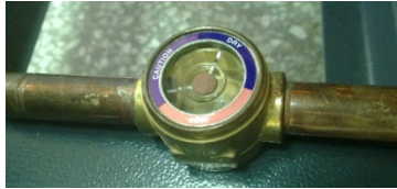
Picture 2-9: Refrigerant Indicator
