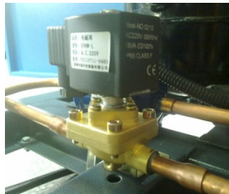
Picture 2-10: Liquid Pipe Solenoid Valve
