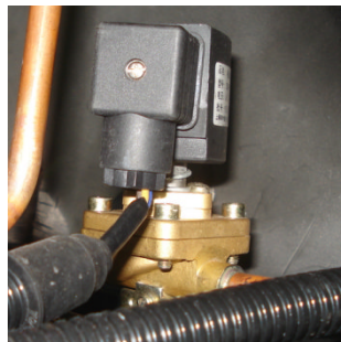
Picture 2-11: Hot-gas By-pass Valve
