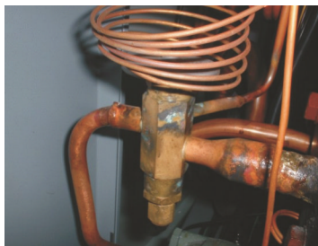
Picture 2-5: Thermal Expansion Valve
