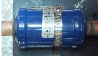
Picture 2-16: Drying Filter
