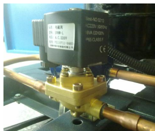
Picture 2-19: Solenoid Valve
