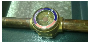
Picture 2-18: Refrigerant Indicator
