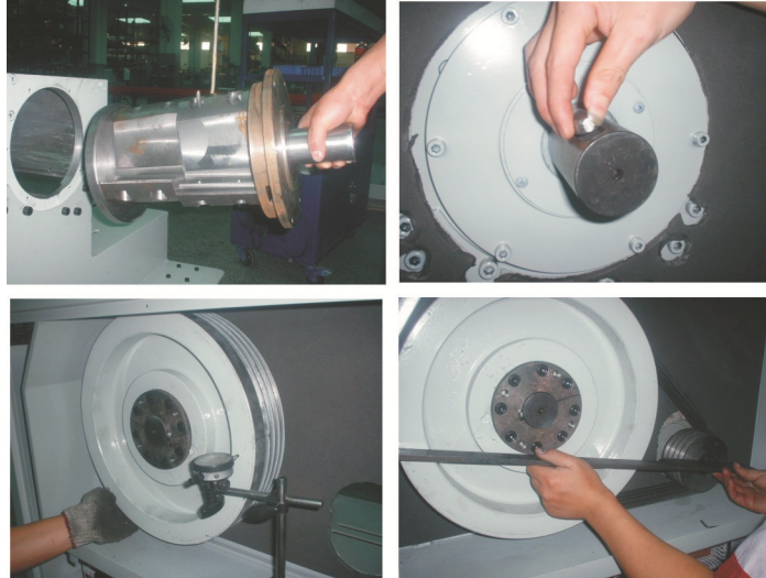
Picture 3-7: Installation of the Bearing, Belt Pulley and Belt
