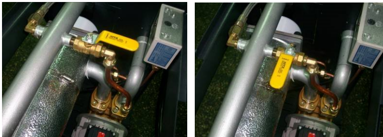
Picture 6-8: By-pass Globe Valve
