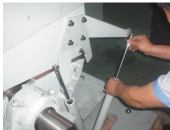
Picture 3-14: Installation of Screen, Screen Frame and Storage Bin 4
