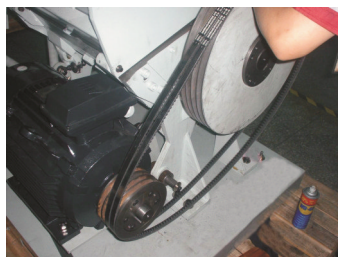
Picture 3-6: Installation of Belt Pulley and Motor 3
