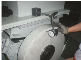
Picture 3-5: Installation of Belt Pulley and Motor 2
