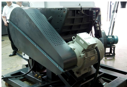
Picture 6-10: Installation of Belt Pulley and Motor 4
