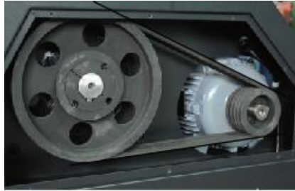
Picture 6-6: Installation of Bearing, Motor, Pulley and Belt
