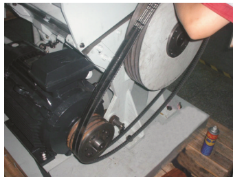
Picture 6-12: Installation of Belt Pulley and Motor 3 (SG-3675)
