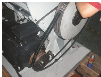
Picture 6-7: Installation of Belt Pulley and Motor 2(SG-3650)
