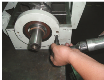
Picture 6-6: Installation of Bearing and Cutter Shaft 3
