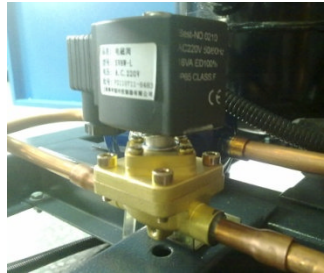
Picture 2-9: Liquid Pipe Solenoid Valve
