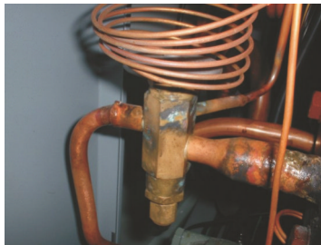
Picture 2-5: Thermal Expansion Valve
