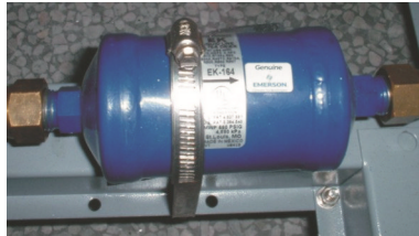
Picture 2-4: Drying Filter
