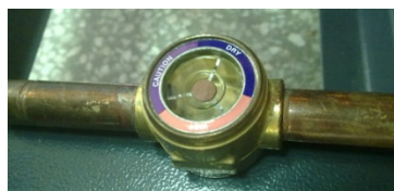
Picture 2-8: Refrigerant Indicator
