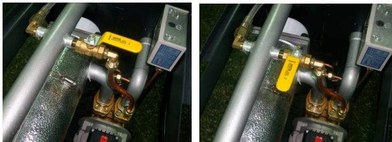
Picture 6-8: By-pass Globe Valve
