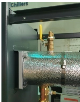
Picture 6-8: By-pass Globe Valve
