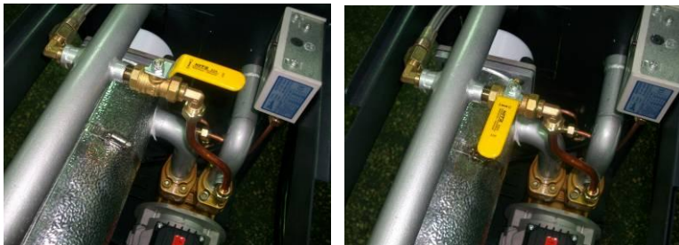
Picture 6-8: By-pass Globe Valve
