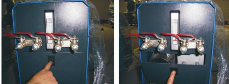
Picture 6-9: Cooling Pipes 1
