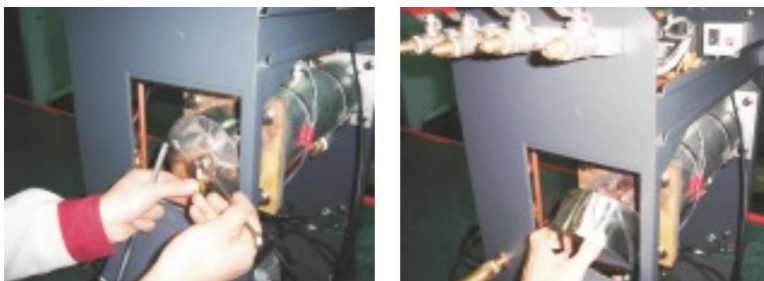
Picture 6-7: Pipe Heater 2
