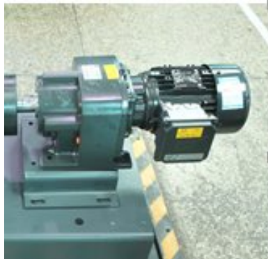
Picture 6-20: Installation of Reduction Gear 1
