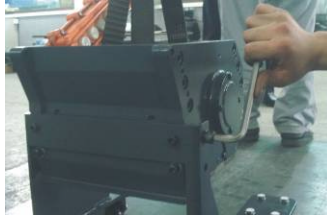
Picture 6-11: Installation of Belt and Belt Pulley 1
