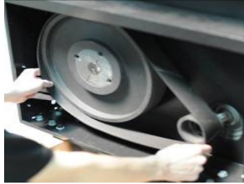
Picture 6-16: Installation of Belt and Belt Pulley 6
