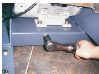
Picture 6-18: Installation of Belt and Belt Pulley 8
