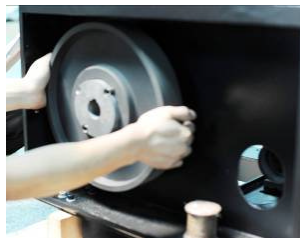
Picture 6-13: Installation of Belt and Belt Pulley 3
