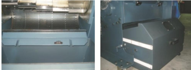
Picture 3-8: Installation of Screen, Screen Frame and Storage Bin.
