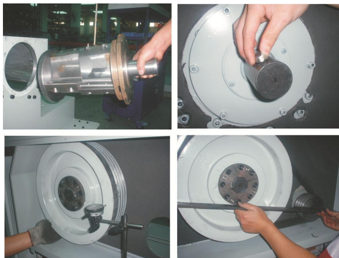
Picture 3-7: Installation of the Bearing, Belt Pulley and Belt
