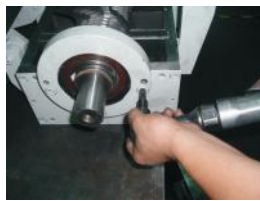
Picture 3-5: Installation of Bearing and Blade Rest 1 3
