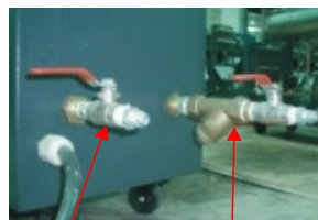
Cooling water outlet Cooling water inlet
