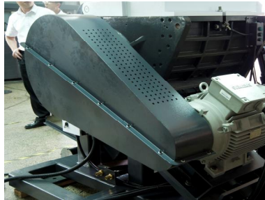
Picture 6-8: Installation of Belt Pulley and Motor 4
