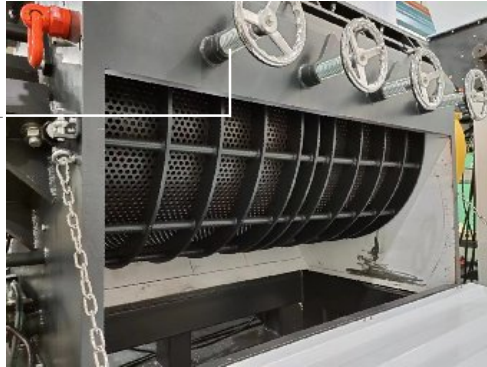
Picture 6-11: Installation of Screen, Screen Bracket and Storage Box 3
