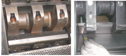
Picture 6-3: Fixed Blade and Rotating Blade Installation
