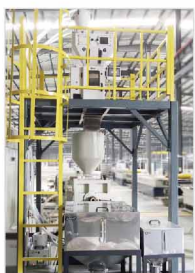
計量混合 Dosing and Mixing
