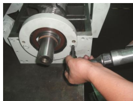
Picture 6-11: Installation of Bearing and Blade Rest 1 3
