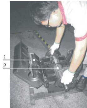
Picture 6-10: Installation of Bearing and Blade Rest 2
