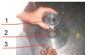
Picture 3-2: Installation of Bearing and Blade Rest
