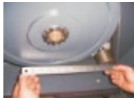
Picture 3-9: Installation of Belt and Belt Pulley 6
