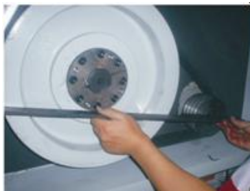
Picture 3-7: Installation of Belt and Belt Pulley 4
