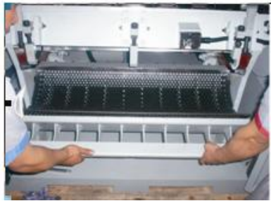
Picture 3-10: Installation of Screen Bracket and Screen
