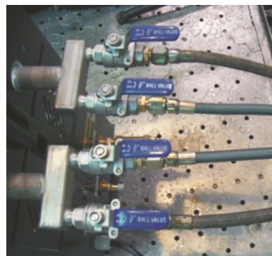
Picture 3-3: Pipeline Connection 2
