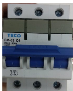
Picture 4-2: Main Power Circuit Breaker
