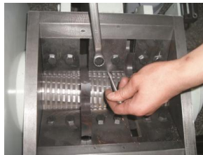
Picture 3-10: Installation of Rotating Blade and Fixed Blade 3
