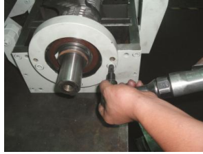
Picture 3-9: Installation of Rotating Blade and Fixed Blade 2
