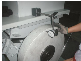
Picture 3-5: Installation of Belt Pulley and Motor 2
