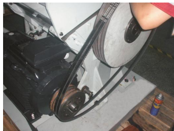
Picture 3-6: Installation of Belt Pulley and Motor 3
