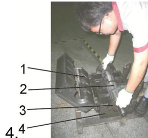
Picture 6-3: Installation of Bearing and Blade Rest 3
