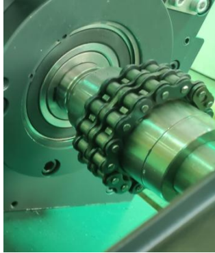
Picture 6-5: Installation of Gear Motor 2
