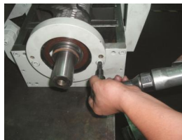
Picture 6-13: Installation of Fixed Blades and Rotating Blades 2
