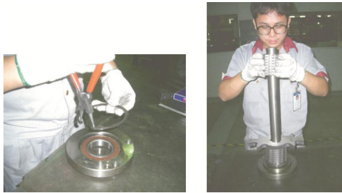
Picture 6-12: Installation of Fixed Blades and Rotating Blades 1
